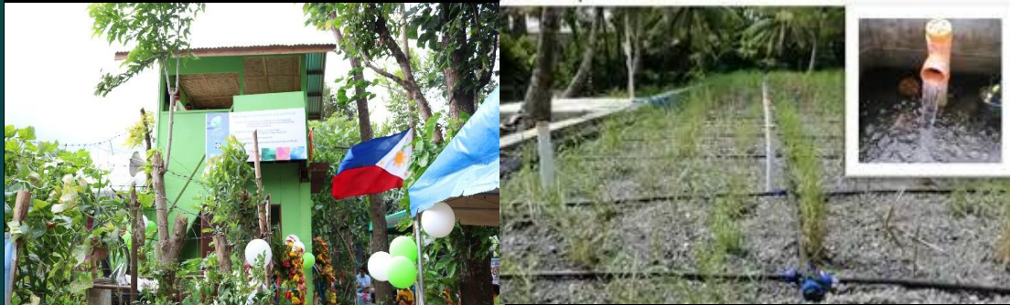
Installation of Vertical Helophyte Filter System and Community Learning Center for DRRM in Davao River Basin
